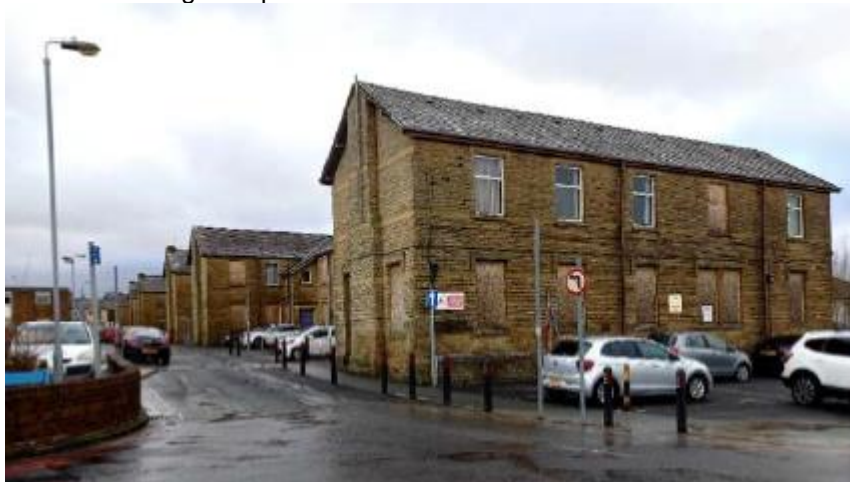
Stone Cottages (photo from submitted Historic Building Survey report)
