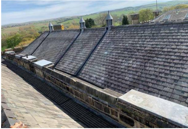
Spine wall between roofs looking east
