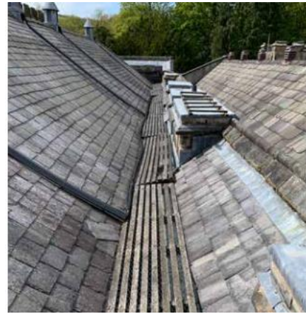
Spine wall looking west
